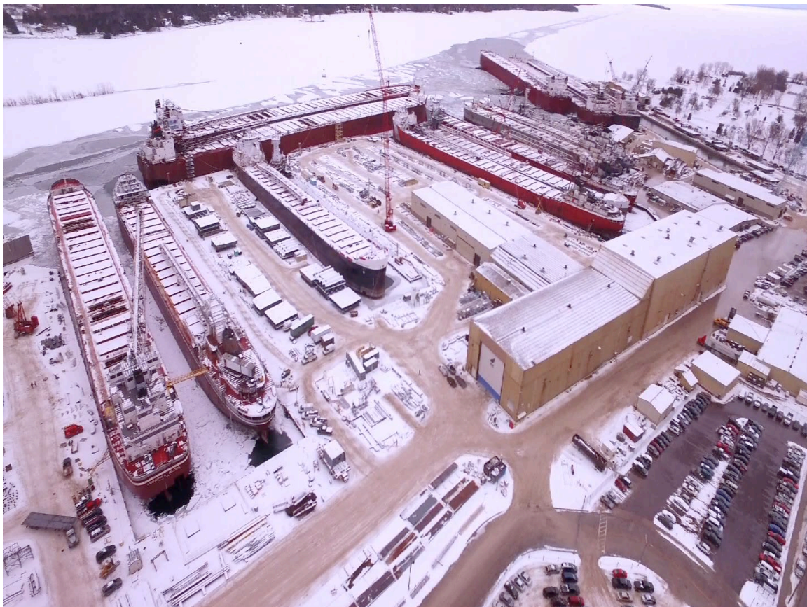
Photo: Recent aerial of Fincantieri Bay Shipbuilding shows 17 vessels of the Great Lakes Bulk Carrier fleet in for Winter repairs.
